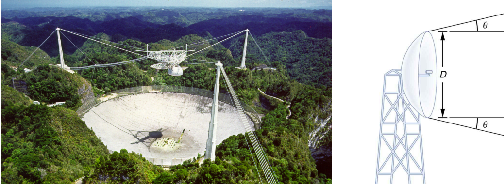
Figure 1: Left: The Aricebo telescope before it was damaged. Credit: NAIC.
